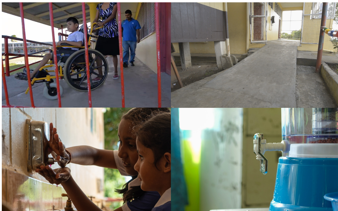
Some examples of suitable WASH infrastructure from schools in Fiji.
